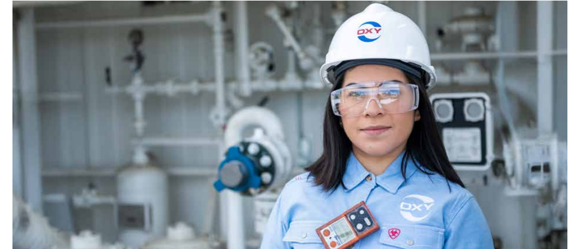
Separation Facility, Platteville, CO
