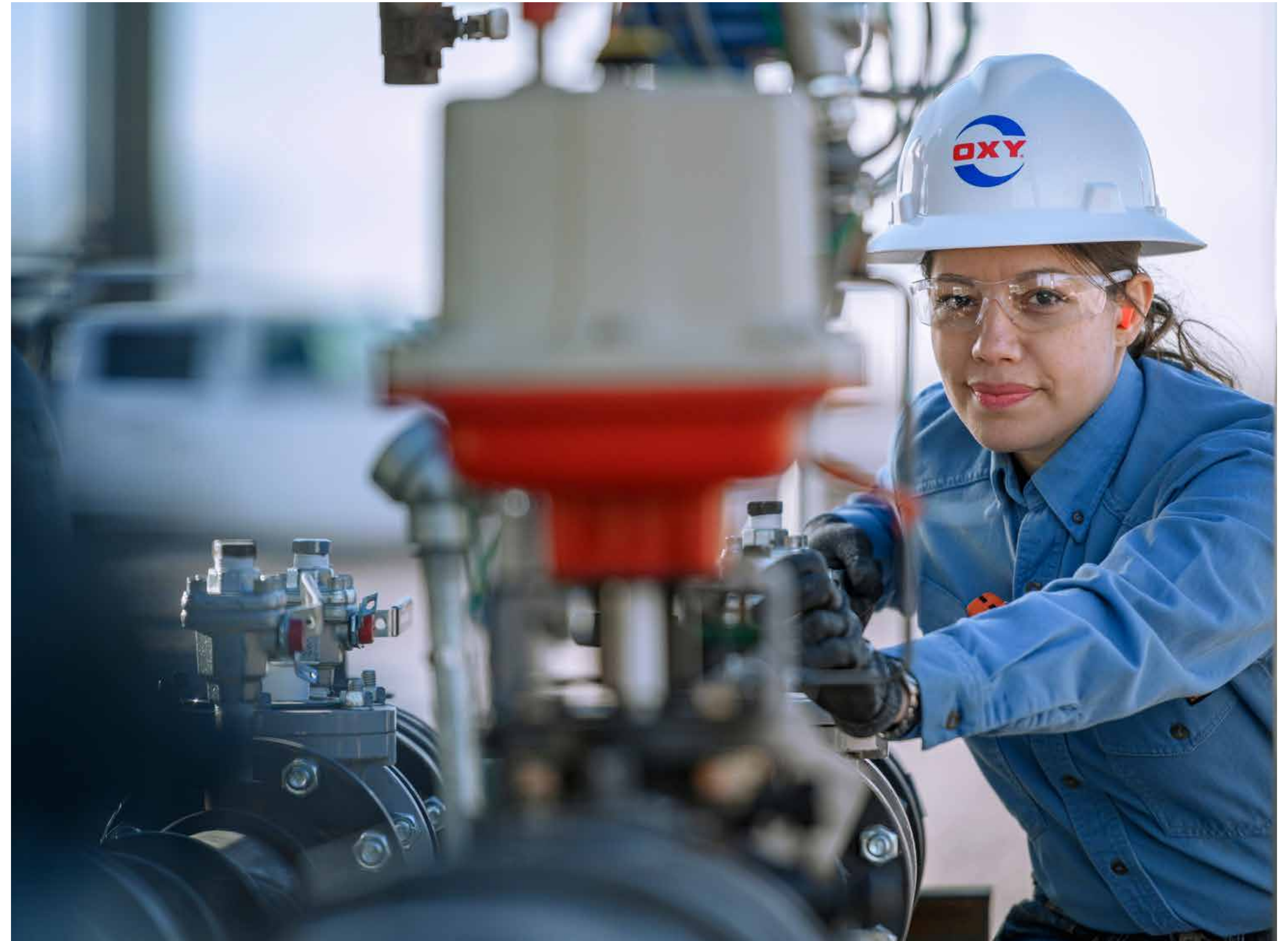
EOR Facility, Hobbs, NM
