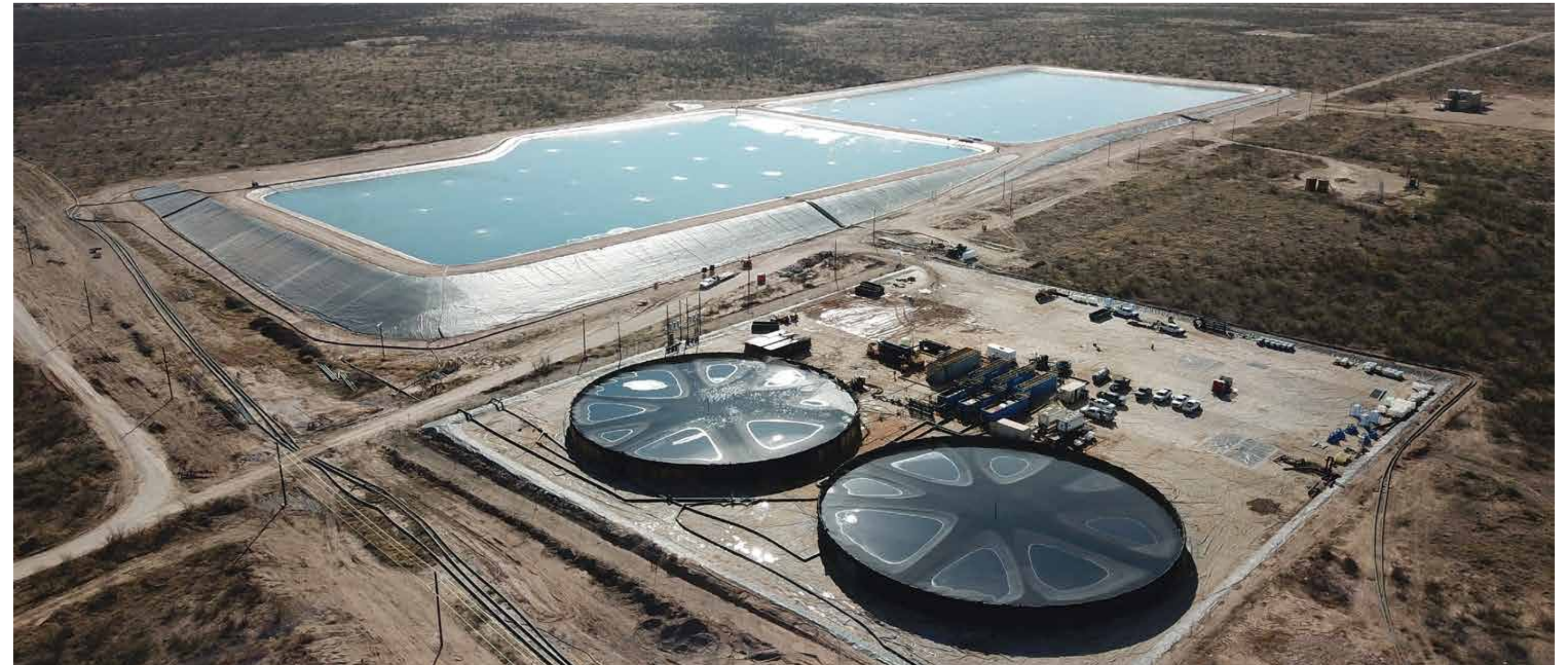
Wrage Produced Water Recycling Facility, Glasscock County, TX
