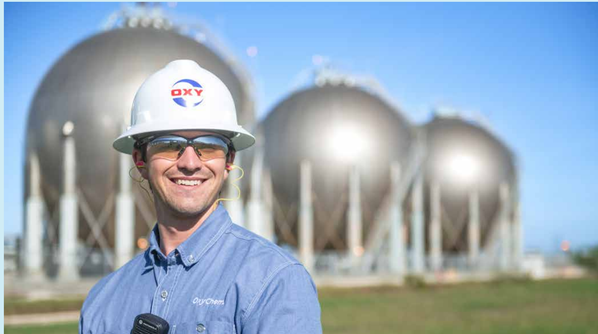
OxyChem Ingleside Plant, TX
