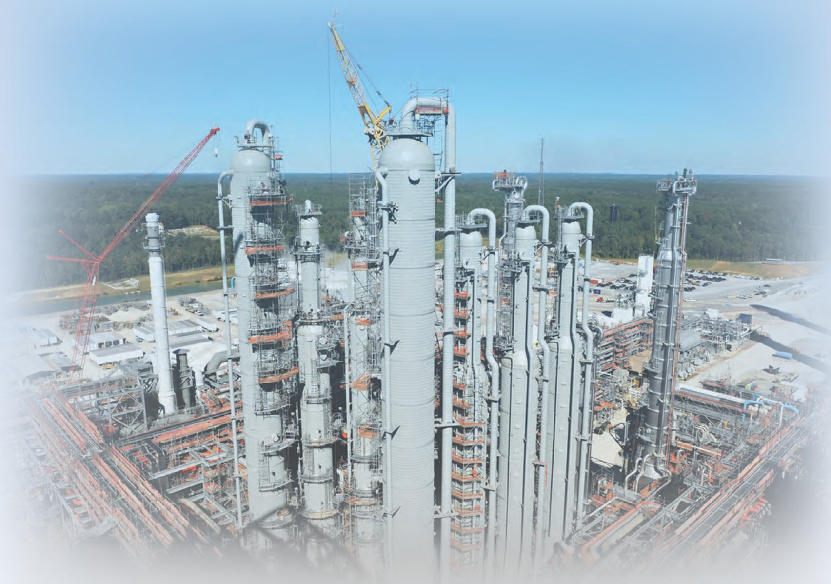
Background image: Scaffolding begins to come off of CO 2 and hydrogen sulfide absorbers at the Kemper County Energy Facility, October 2014. All rights reserved by Mississippi Power's Kemper County Energy Facility.
