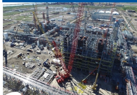
INGLESIDE - ETHYLENE CRACKER
